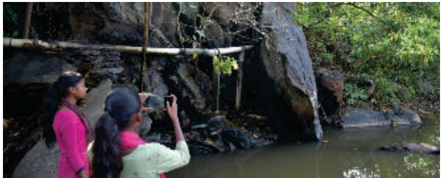
Pipeline constructed to collect stream water
