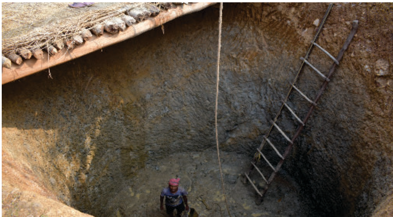
Construction of well to collect rain water
