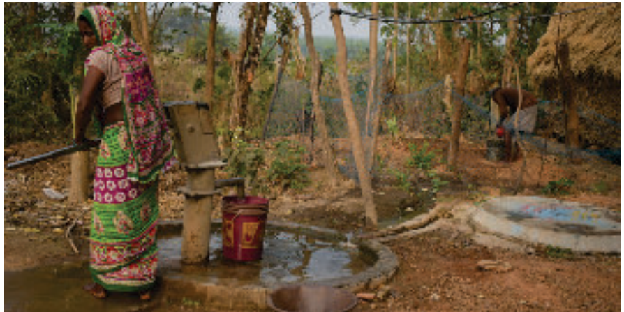
Pit has been constructed in front of tube wells to collect waste water
